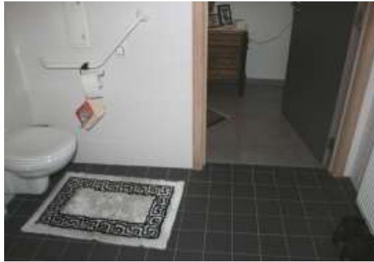
toilet in badkamer
